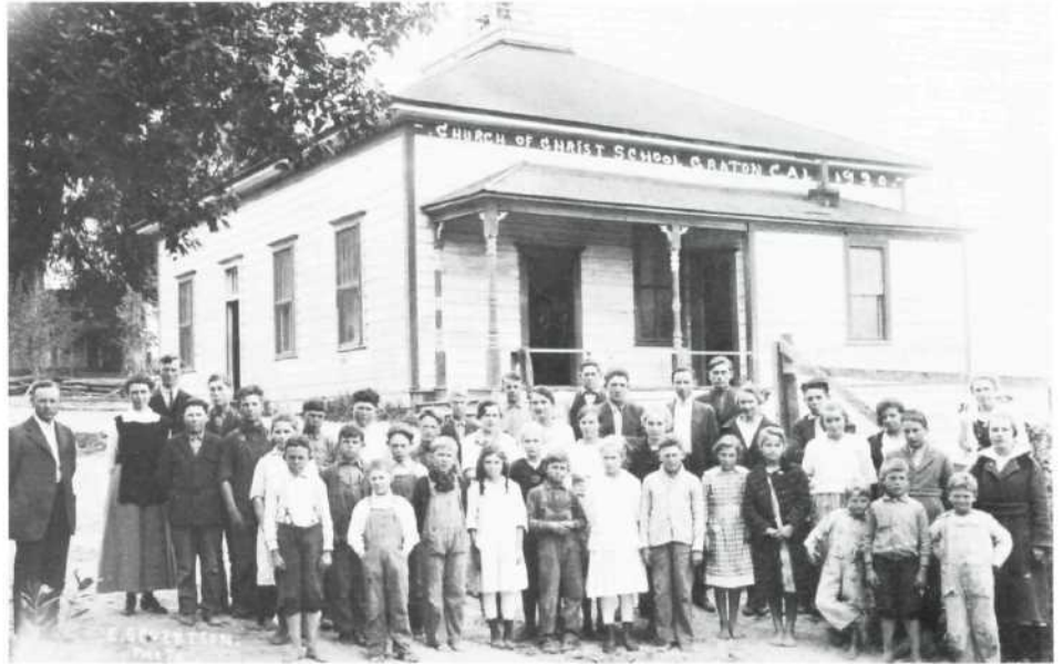
In the second year of operation, P.C.A. moved into this 3-room school building in Graton.
