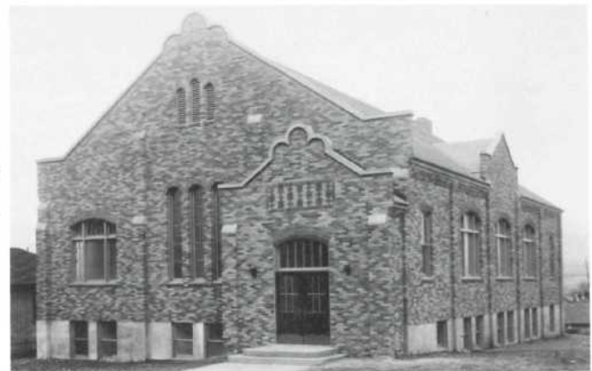
Constructed in 1930 and later expanded, the Okanogan Avenue building served the church for 58 years.
