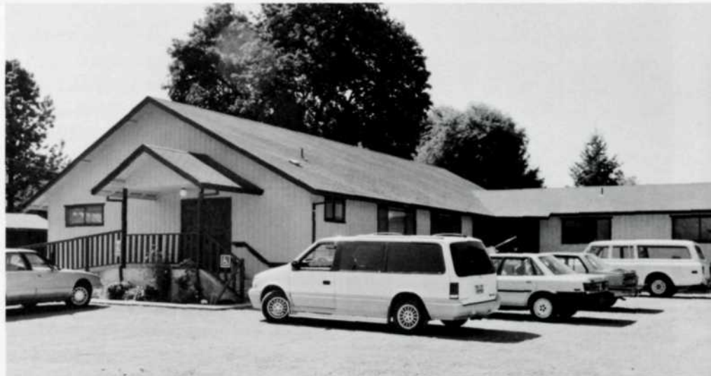
The Tri-City Church's building, erected in 1980, received a classroom wing about five years ago. Increasing attendance has made two Sunday services necessary.
