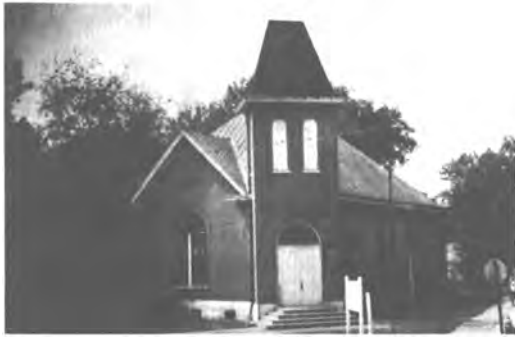
Reid Avenue Church of Christ, Nashville, Tennessee
